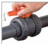
Nuts tightening
